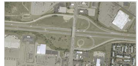
The original interchange did not provide adequate capacity and impeded the flow of traffic.
