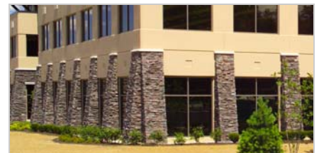
For architectural interest around the building perimeter, stone accents were applied to tapered concrete buttresses.
