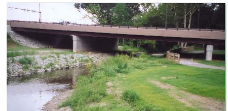
The bikeway was relocated to create a more scenic path and remove a dangerous crossing on North Fairfield Road.
