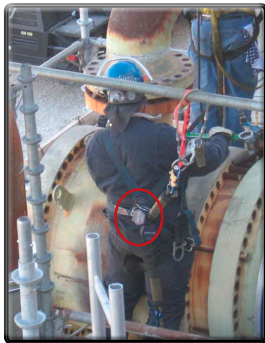
Photo 1: In this example, the back-mounted SRD has slid down to hip level, rather than being in between the shoulder blades as required for proper use.
