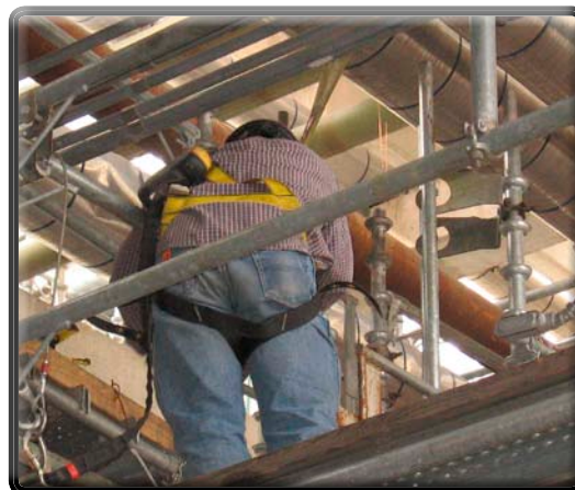
Photo 3: In this configuration, excess free fall would occur as a result of anchorage at foot level.
