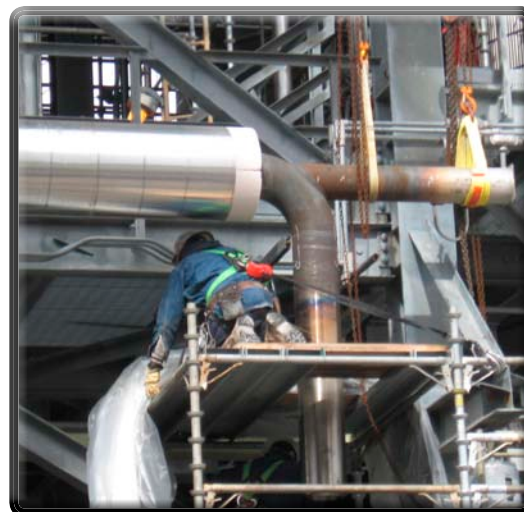
Photo 2: It is critical to plan for fall protection equipment use so that anchorages can be located overhead, rather than away from the body at foot level.
